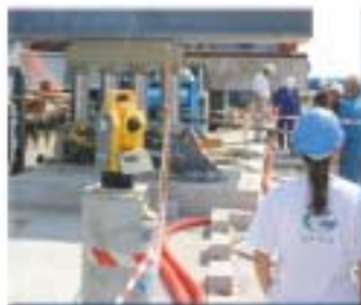
GEOID employed a team of 9 surveyors to position the main breakwater
